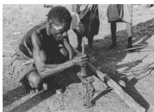
The bar ( Museya ) meant to be wire-drawn is passed through the drawing die through a hole in the lever-beam and is gripped by the vise ( Muganga ). 1956, Katanga, RDC. HPI 1984.25.69-24, collection RMCA Tervuren; photo UMHK, 1957, RMCA Tervuren © Graphic L. G.-Marot
