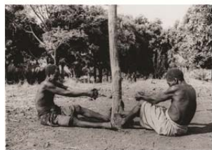
Drawing of a wire less than 2mm thick, the kwebele, at the village of Nguba, 1956, Katanga, DRC. HP1984.25.69-20, collection RMCA Tervuren; photo UMHK, 1957, RMCA Tervuren © Graphic L. G.-Marot
