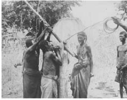
Chief Nguba observing the correct positioning of the lever. Behind the lever is the vise, the Munganga , which hold the copper bar, the Museya . The copper bar runs through the lever and the drawing die. Village of Nguba, 1924, Katanga, DRC. HP1194.25.69-47, collection RMCA Tervuren; unknown photographer, 1924 © Graphis L. G.-Marot
