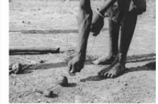
Setting the wire and the die for drawing the Nsambo. Village of Ngaba, 1956. Katanga, DRC. HPI 1984.25.69-26, collection RMCA Tervuren; photo LPHMK, 1957, RMCA Tervuren © Graphic L.G.-Marot
